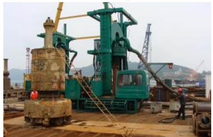
The Hangzhou bay bridge 2.5-2.8m × 128m
