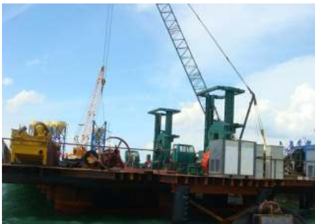
The Penang Second bridge 2.0-2.3m × 115m
