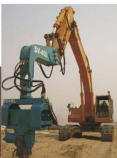
深圳机场工地 working in ShenZhenAirport
